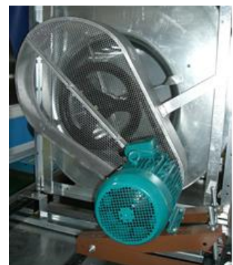
Figure 8: Fan - Motor Assembly
